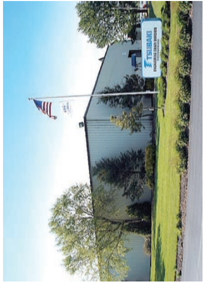
Engineering Chain Plant - Sandusky, OH
